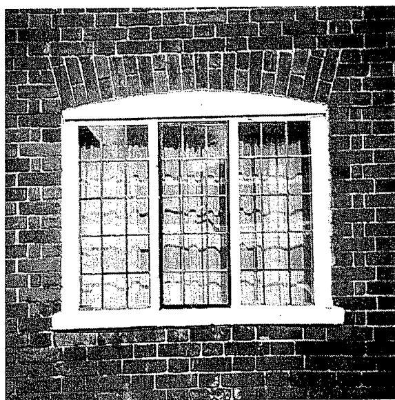
Old windows are part of an area's character and scale
