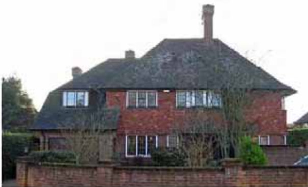
◀ Hollycroft, E Thorpe Close, designed by Robert Muir in 1928, with his trademark wide sprocketed eaves, tile-hanging and corbelled chimneys.
